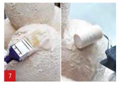
This mixture can be applied with a brush or roller.
