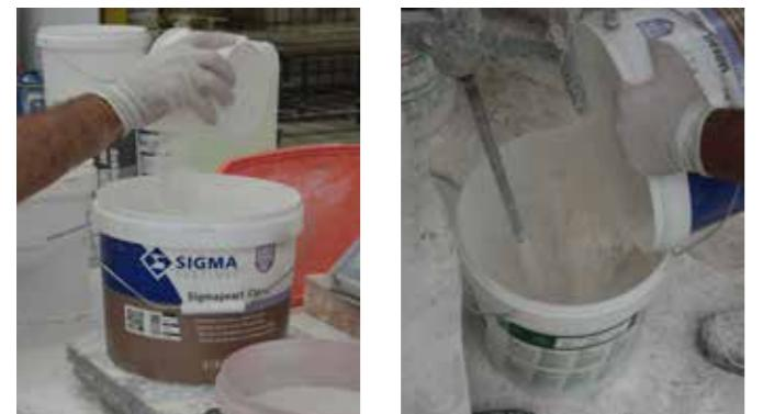
Weighing and mixing A1 Liquid, A1 Powder, Thix A and sand for the top layer.
