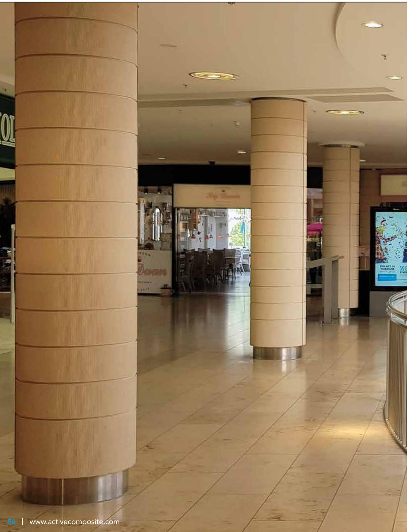
Columns were made by using a mould. A1 was mixed with yellow sand reinforced with several layers of A1 Triaxial fibre.
