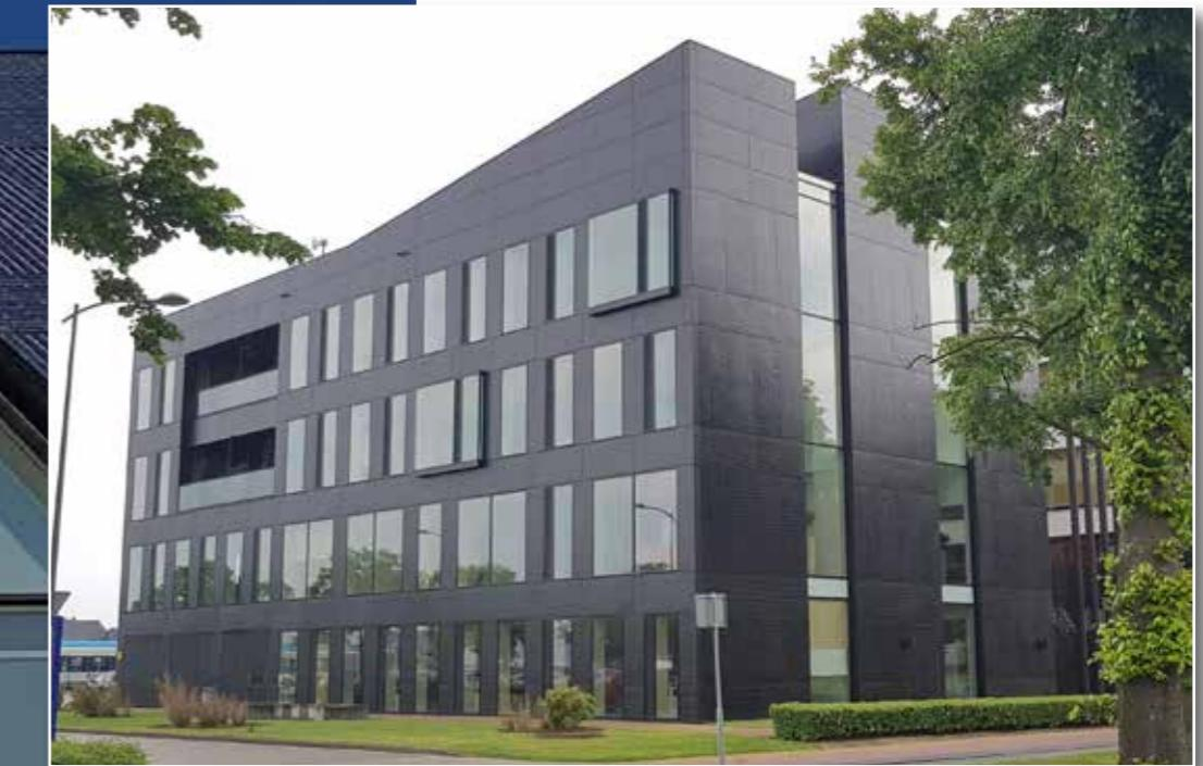
The original façade of this building was damaged badly by weather influence to such an extend that decided was to replace the whole façade. The original feel and look of the façade were to be maintained without the use of the original materials.
