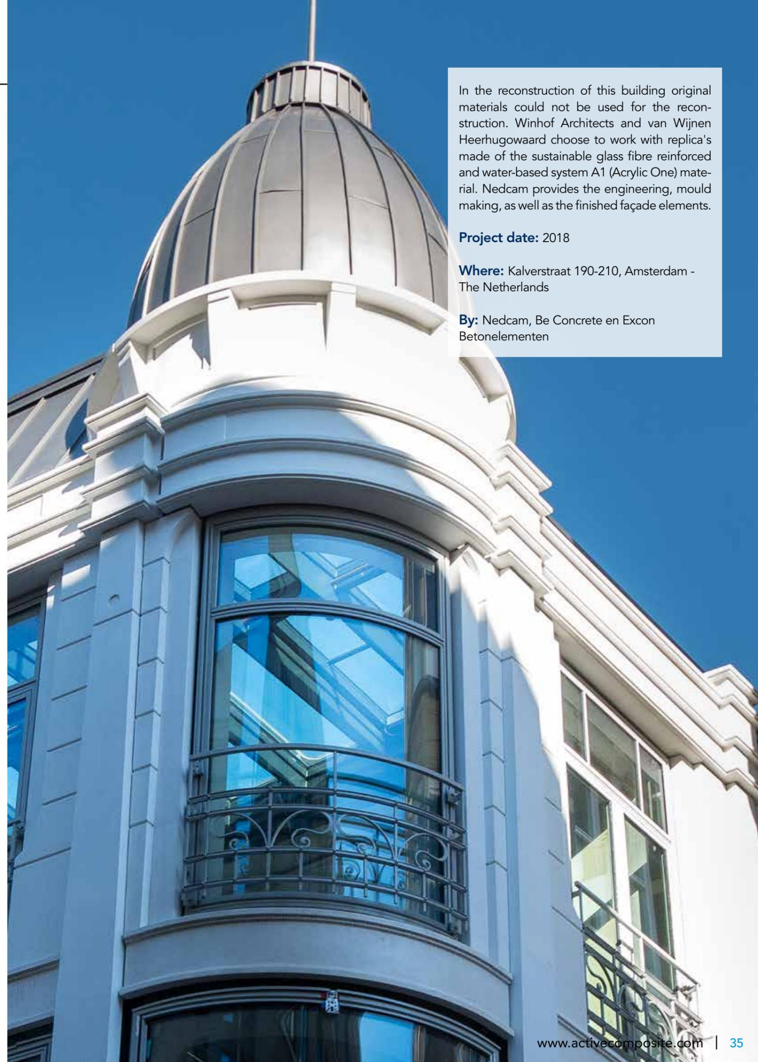
In the reconstruction of this building original materials could not be used for the reconstruction. Winhof Architects and van Wijnen Heerhugowaard choose to work with replica's made of the sustainable glass fibre reinforced and water-based system A1 (Acrylic One) material. Nedcam provides the engineering, mould making, as well as the finished façade elements.
