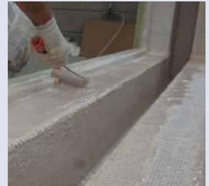
To laminate, you have to work wet in wet. A quick way to apply A1 is with a brush or roller.
