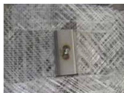
Stainless steel brackets are mounted on the panel.
