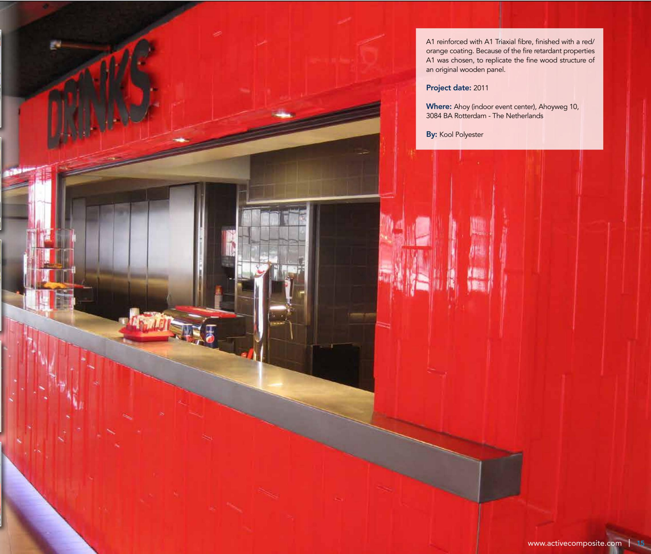
A1 reinforced with A1 Triaxial fibre, finished with a red/orange coating. Because of the fire retardant properties A1 was chosen, to replicate the fine wood structure of an original wooden panel.
