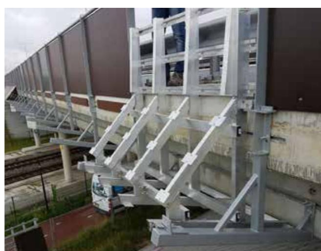
Aluminum structure mounted to the steel structure (without A1 element)
