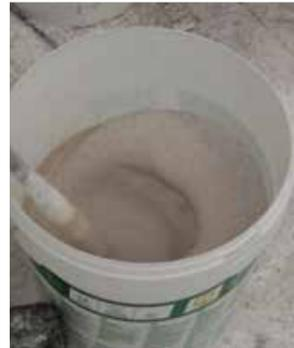
Weighing and mixing A1 Liquid, A1 Powder, Thix A and sand for the top layer.
