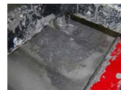
The stainless steel brackets were embedded with A1 with chopped glass fibres.
