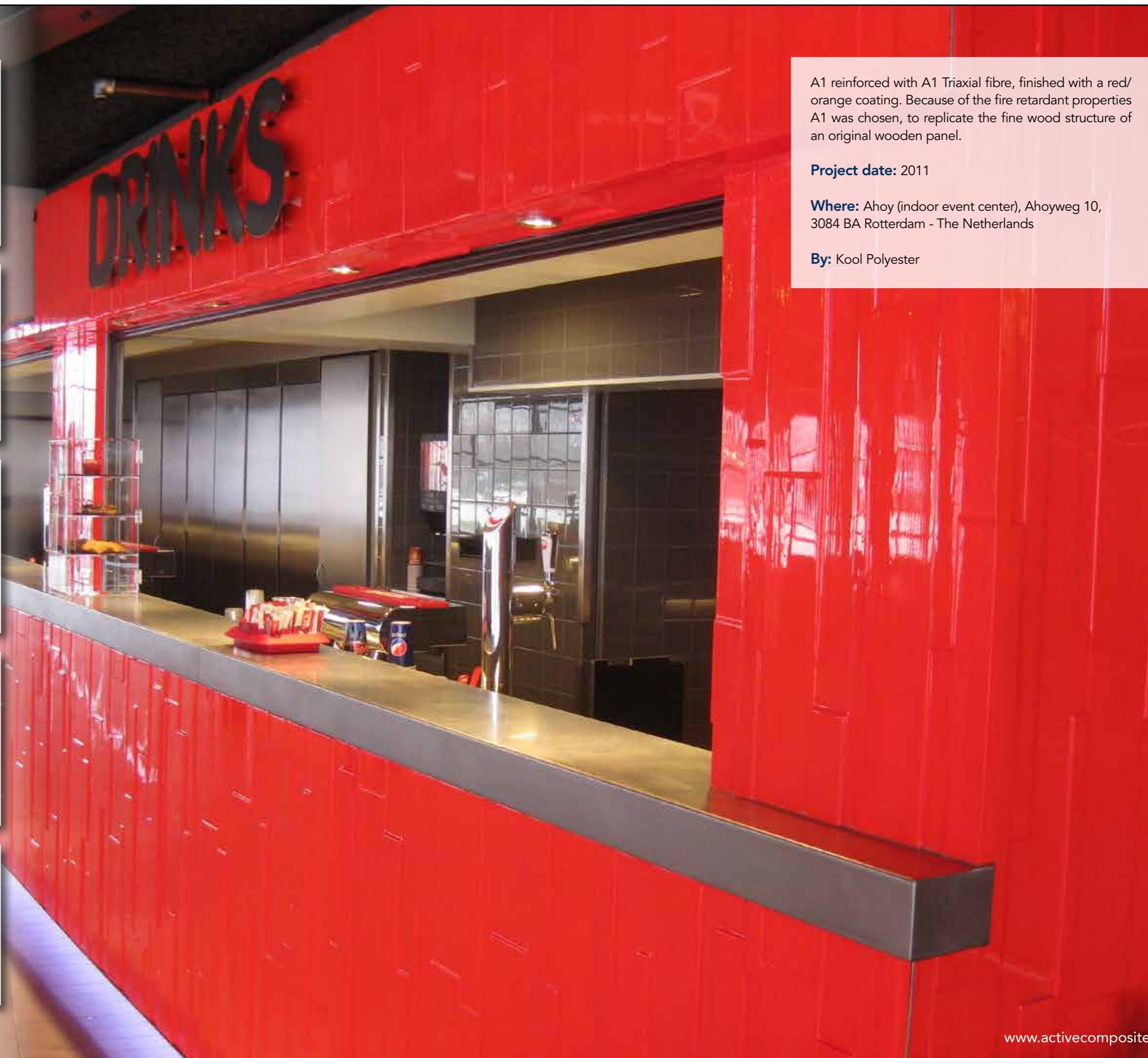
A1 reinforced with A1 Triaxial fibre, finished with a red/orange coating. Because of the fire retardant properties A1 was chosen, to replicate the fine wood structure of an original wooden panel.
