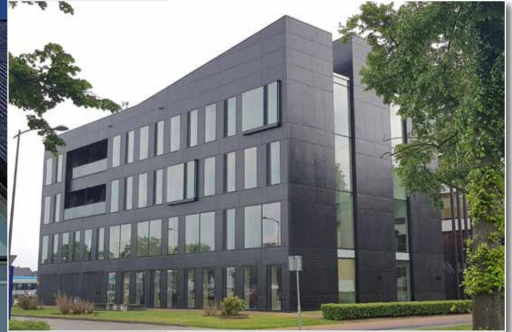
The original façade of this building was damaged badly by weather influence to such an extent that it was decided to replace the whole façade. The original feel and look of the façade were to be maintained without the use of the original materials.
