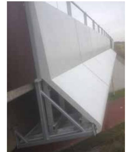
The final result is a bridge edge built up from elements that are accurately aligned. A concrete look is realized by using A1 that has 80% less weight than a bridge edge that would be made of concrete.
