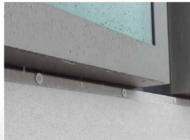
In order to avoid accumulation of moisture due to condensation, an opening is created between the element and the building structure.
