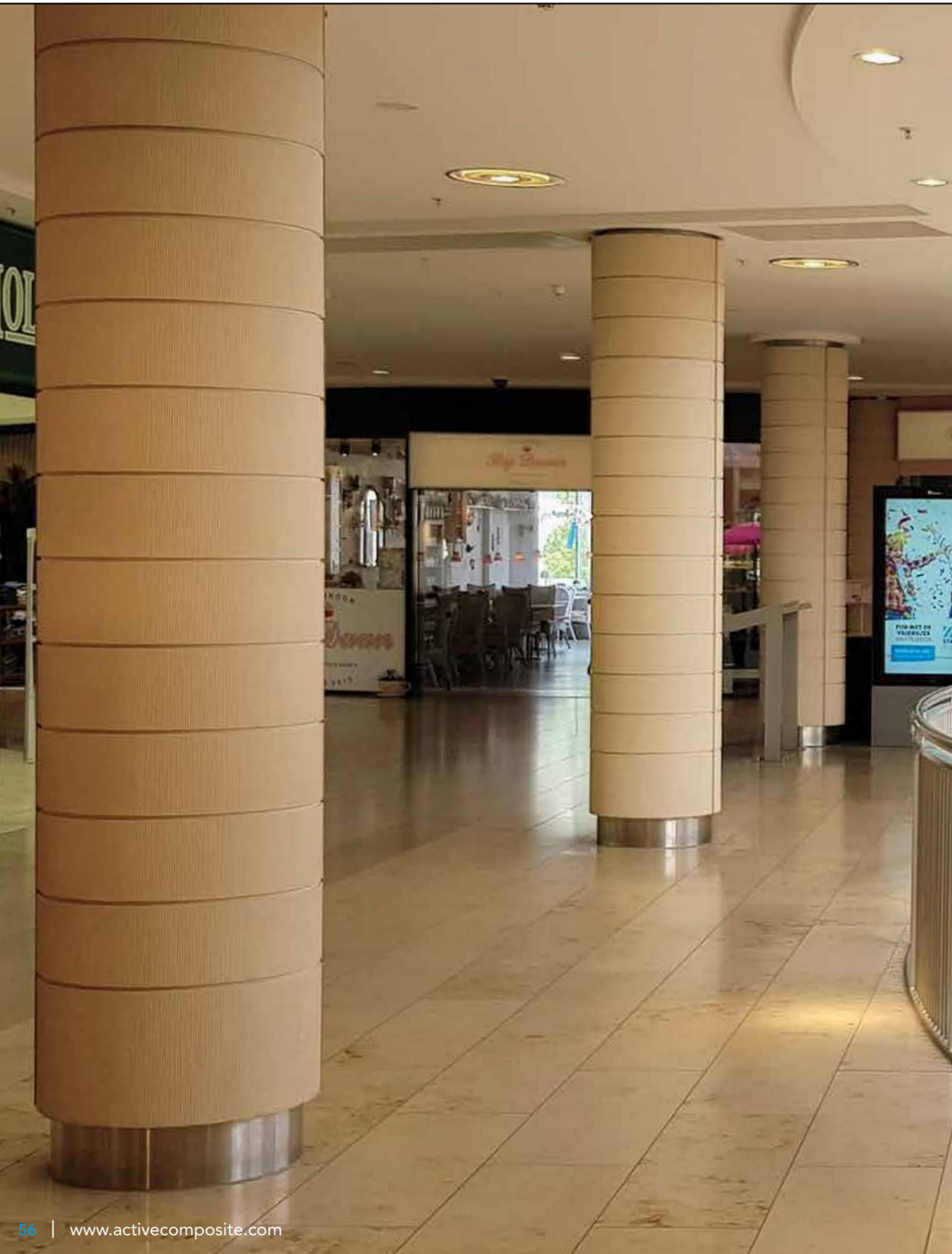
Columns were made by using a mould. A1 was mixed with yellow sand reinforced with several layers of A1 Triaxial fibre.
