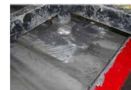
3 layers of A1 Triaxial fibre is laminated on the brackets to get a strong connection.
